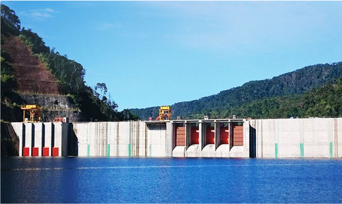
Xekaman 1 powerhouse and tailrace image below:
