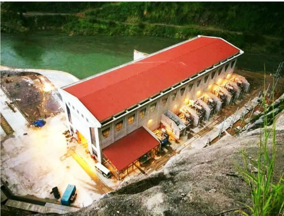
Xekaman 1 powerhouse rotor installation image below:
